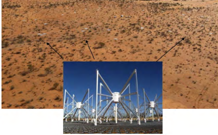
Figure 2: Aerial photograph of the MWA site in Western Australia, showing the first 32 deployed tiles and (inset) a close up of an antenna tile consisting of 16 dipoles placed on a ground screen (Lonsdale et al., 2009).
