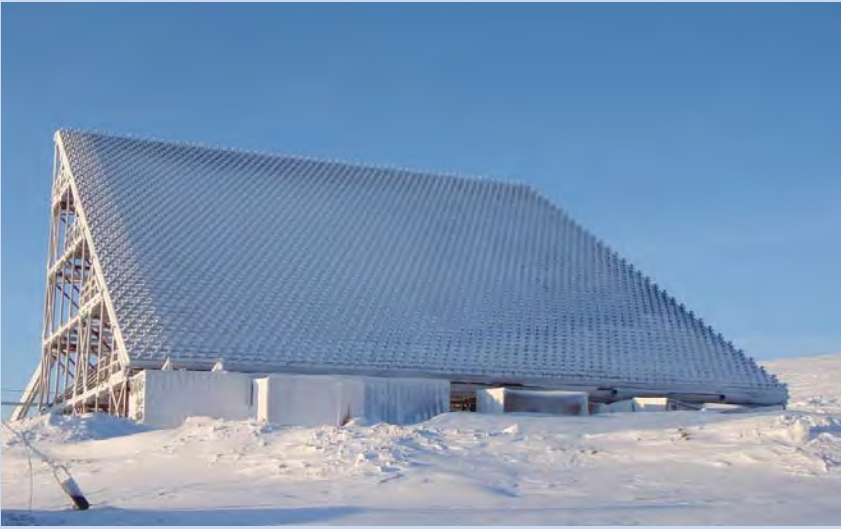
Figure 4: Resolute Bay, Canada: The Advanced Modular Incoherent Scatter Radar provides continuous, reliable, unattended, and autonomous operation delivering high time resolution, high precision ionospheric profiles and imaging under all conditions in real time. The modular construction uses commercially fabricated units to achieve low initial capital investment, fault tolerant and efficient operations, and reduced maintenance costs. (Photo: Craig Heinselman)
