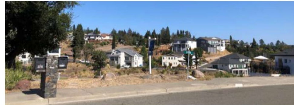
Rebuilding progress in affluent WUI areas, Sept 2022
