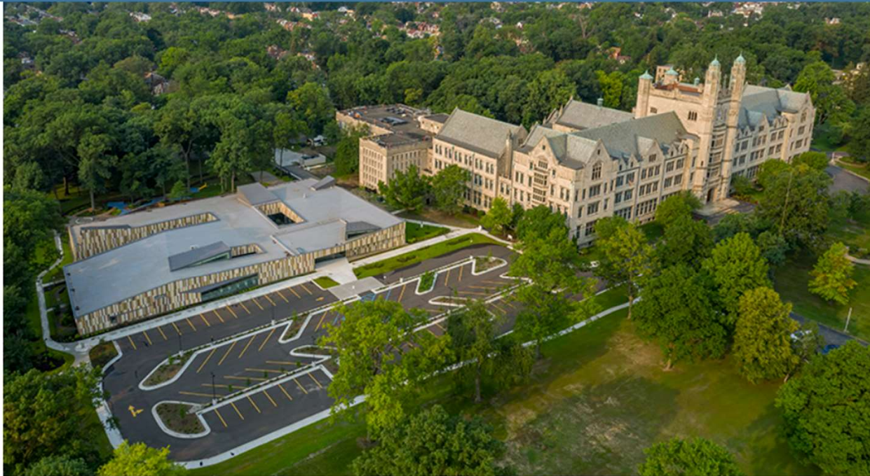
The Marygrove Early Education Center was designed to harmonize with existing campus buildings, particularly the Liberal Arts Building erected in 1925. (Photo: Timothy Hursley copyright)
