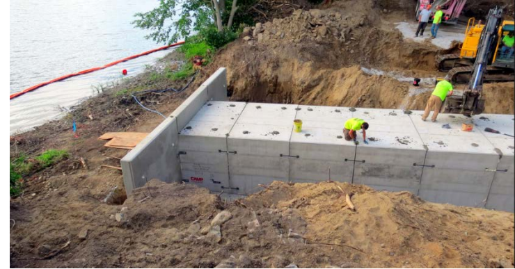
Enlarging culvert in Vermont after Hurricane Irene in August of 2011
