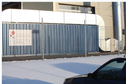
GPAO pollution control at windmill blade factory
