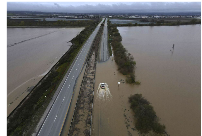
Pajaro River Levee Failure, California 2023
