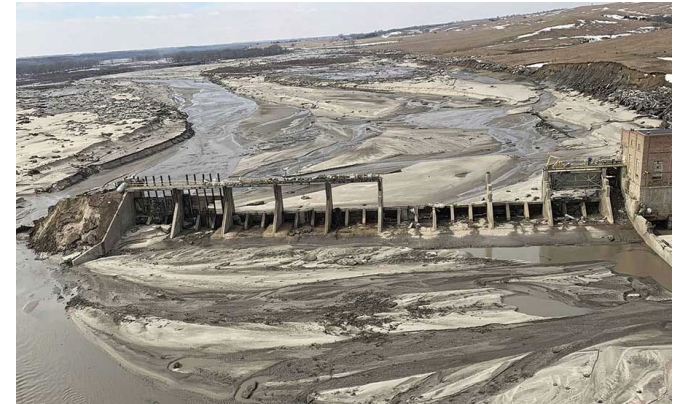
Spencer Dam Failure, Niobrara River Nebraska 2019
