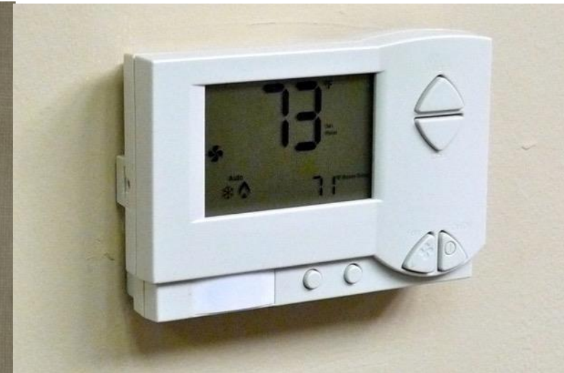
Occupancy activated thermostat
