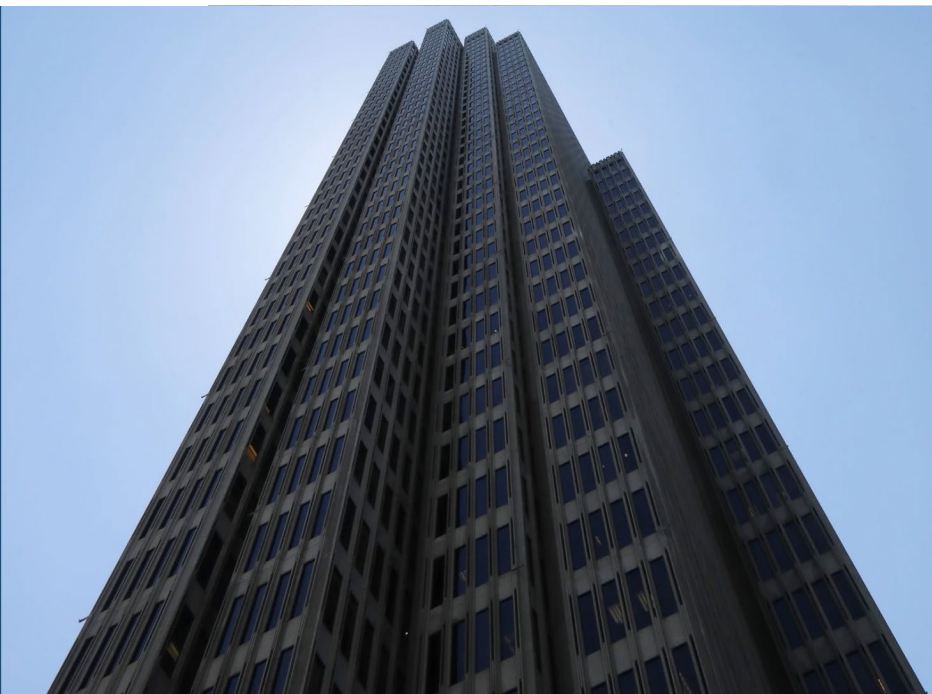
One Embarcadero Center and Two Embarcadero Center in San Francisco. Both are steel-frame buildings, constructed at a time when a flawed welding technique was widely employed. Jim Wilson/The New York Times
