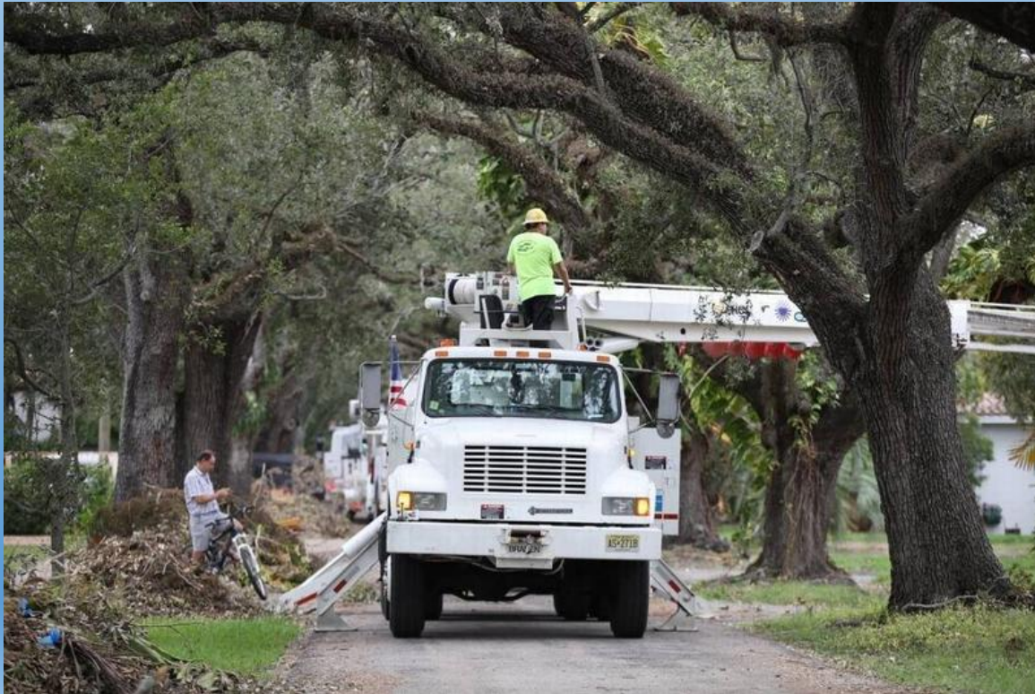
Linemen repair distribution lines in Hurricane Irma (Miami Herald)
