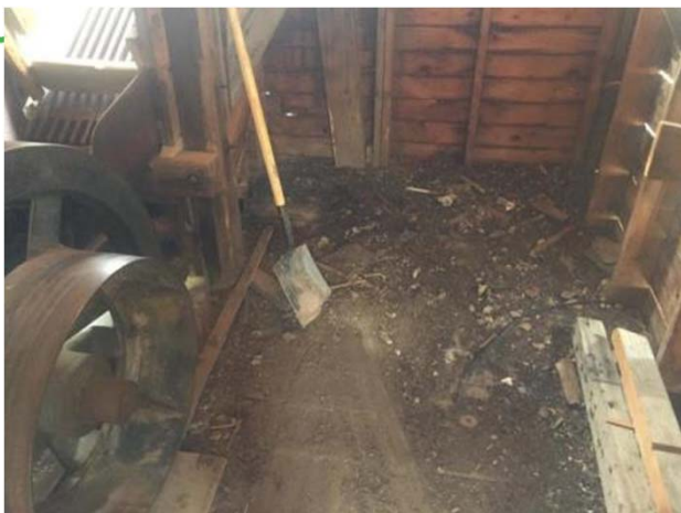
Clean-up and decontamination of Mill building interior
