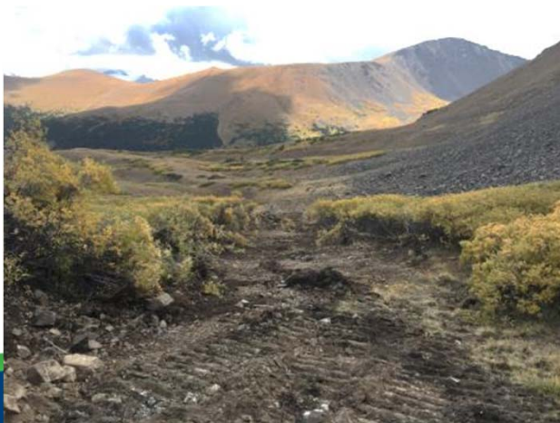
Construction of 600ft run-on-off channel
