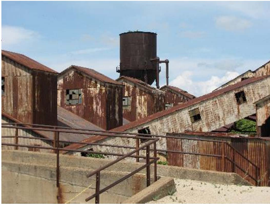
Stabilize buildings at St. Joseph, MO Lead mine
