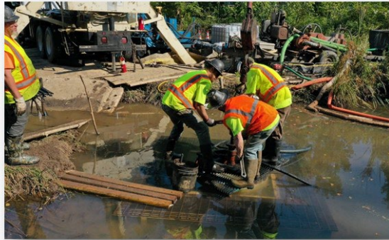
Conductor casing being set and wellhead installed for well control. Photos courtesy of Ohio Dept. of Natural Resources, Division of Oil & Gas Resources Management.
