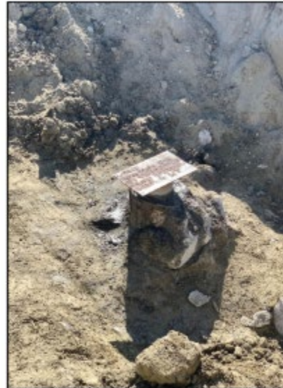
Cut and Cap – Plate welded on
