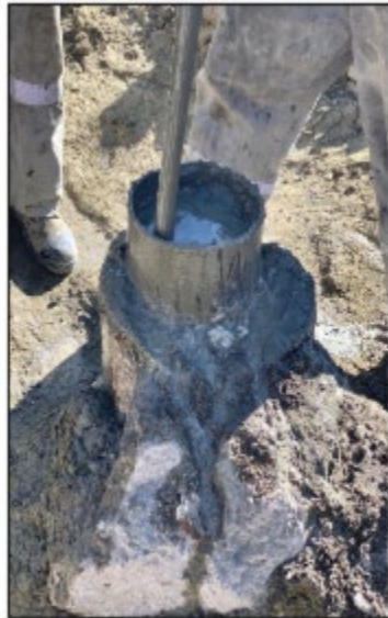
Pumping the surface plug
