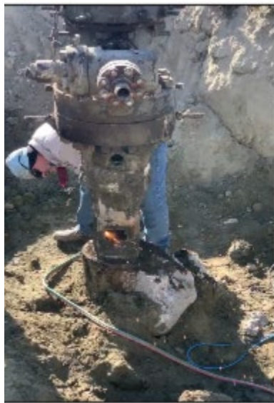
Cutting the well head off
