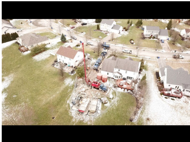
Orphan well in an urban location with very close proximity to neighboring property. Photo courtesy of Ohio Dept. of Natural Resources, Division of Oil & Gas Resources Management.
