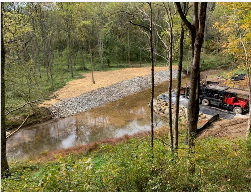
Prior to plugging, the pad was constructed and a cellar ring was constructed for containment. The pad needed to be large enough for the rig and for the pipe trailer. Photo courtesy of Ohio Dept. of Natural Resources, Division of Oil & Gas Resources Management.
