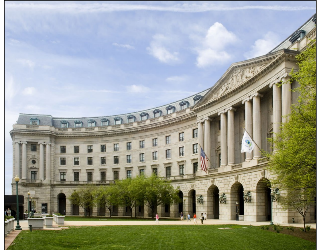
EPA Headquarters in Washington, DC
