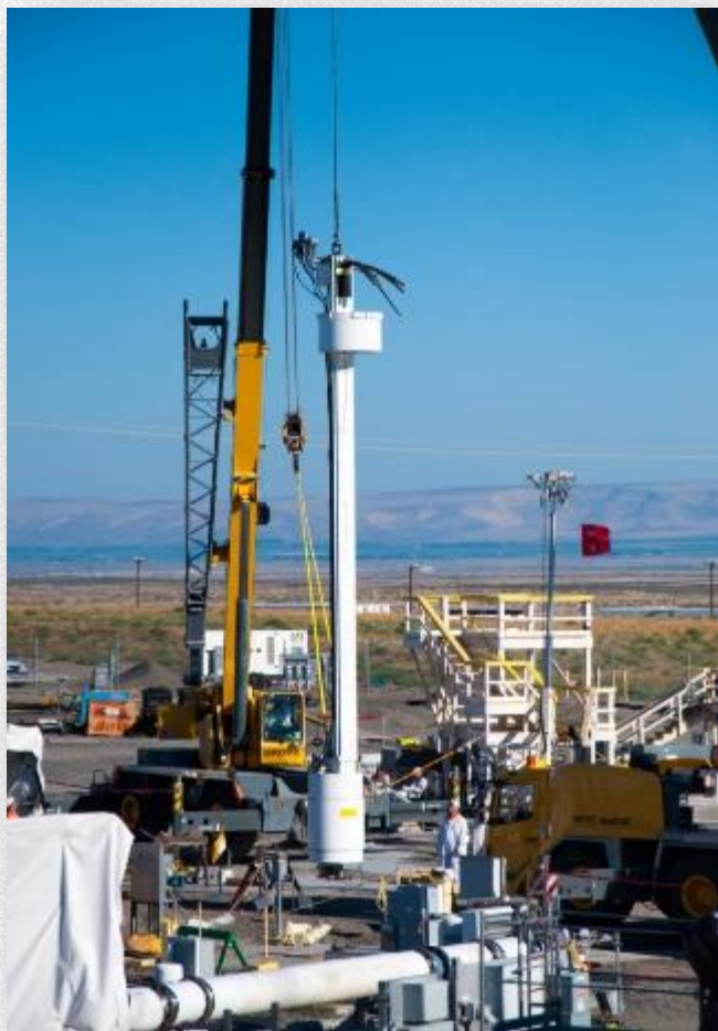
Mast of the MARS-V installed at tank C-105
