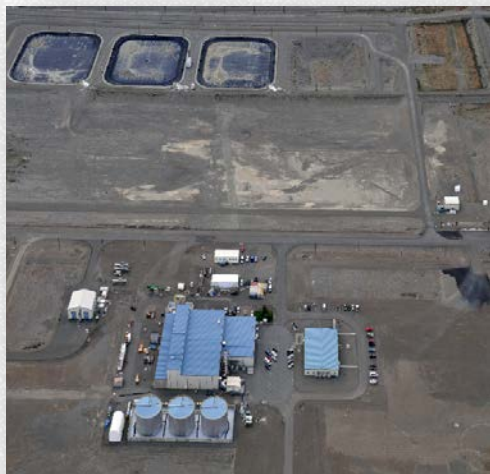
Effluent Treatment Facility
