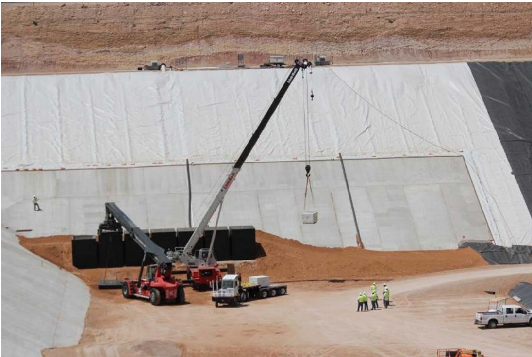
Figure F-18 Wastes being Loaded into Rectangular MCCs inside a Disposal Cell with Components of the Multi-Barrier Liner Visible in the Background (Note the scale of the disposal cell)
