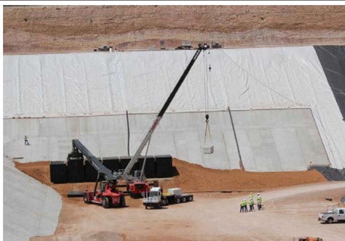
Figure 5-2 A Waste Control Specialists Disposal Cell and Wastes Being Placed in Modular Concrete Canisters (note workers for scale)
