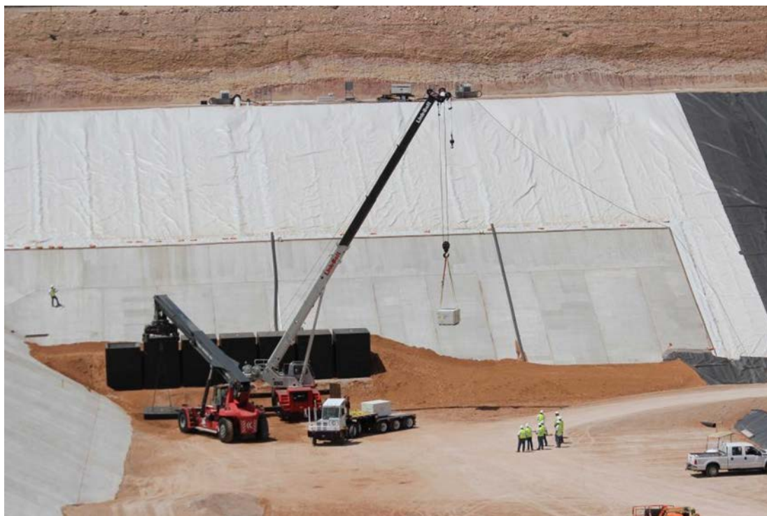
Figure G-3 Wastes being Loaded into Rectangular MCCs inside a Disposal Cell with Components of the Multi-Barrier Liner Visible in the Background (Note the scale of the disposal cell)
