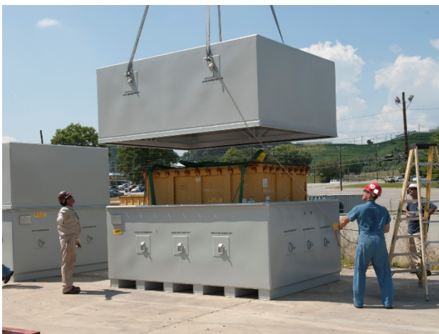
Figure G-3 Example of a Reusable Steel Split-Cavity Overpack (actual overpack would be smaller, lighter, and with a shallower lid) (photograph from Container Technologies Industries, LLC literature 122 )
