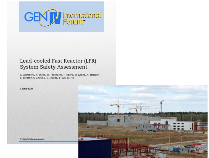
Site preparations for the BREST-OD-300 construction
