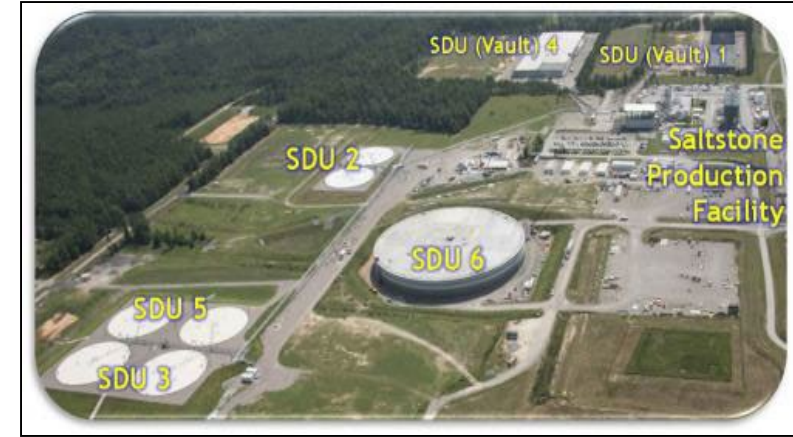
Arial View of Saltstone Disposal Units
