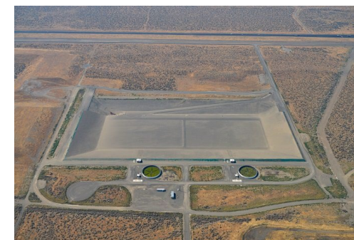
Hanford Integrated Disposal Facility, WA
