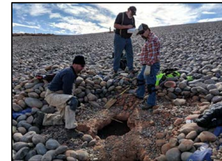
Erosion beneath riprap rock cover at Mexican Hat, Utah
