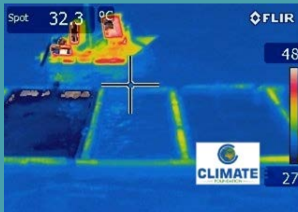
Thermal image of the troughs
