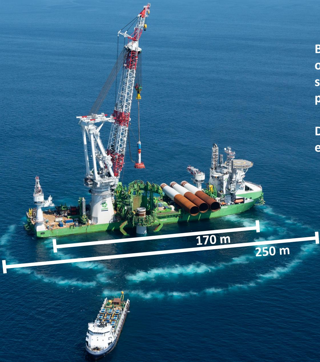
**Bubble curtains are used during installation of monopile foundations to attenuate sound, thereby reducing noise impacts for protected species & fish**
