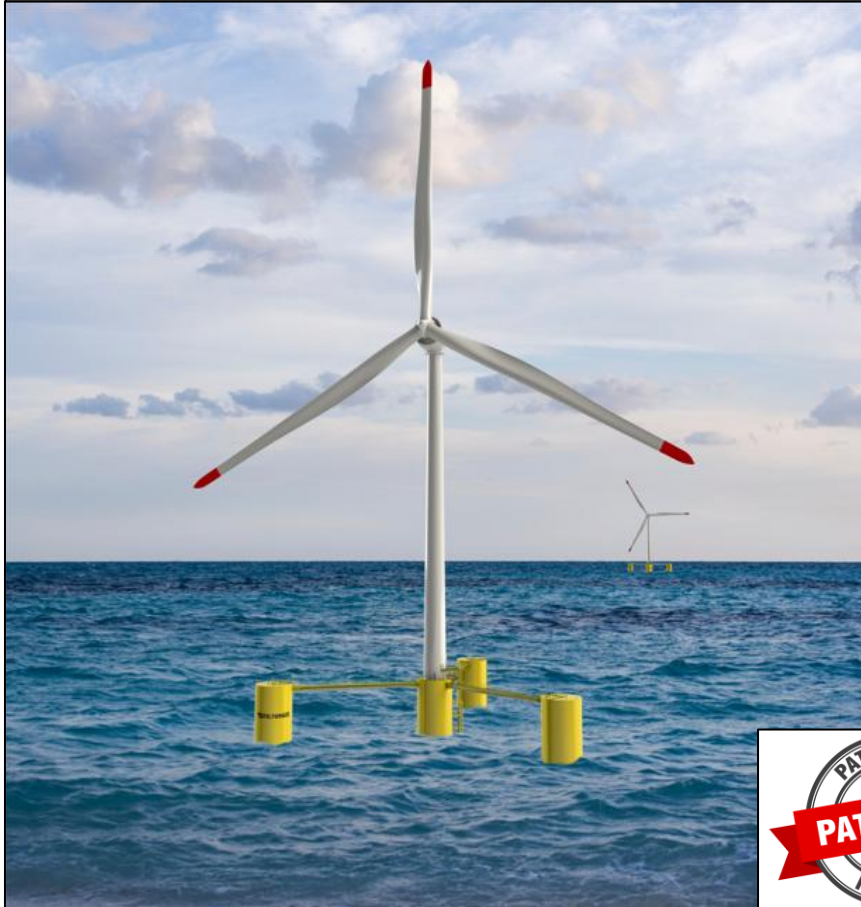
VoltturnUS 4-column concrete semi-sub 1:8 Scale deployment (2013), Catenary chain mooring
