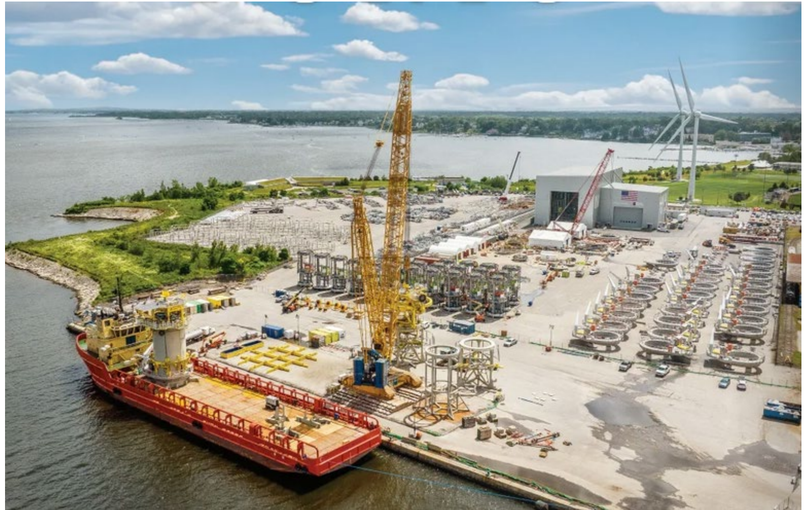
Riggs Distler Advanced Foundation Components for Orsted's Revolution Wind project. ProvPort, RI
