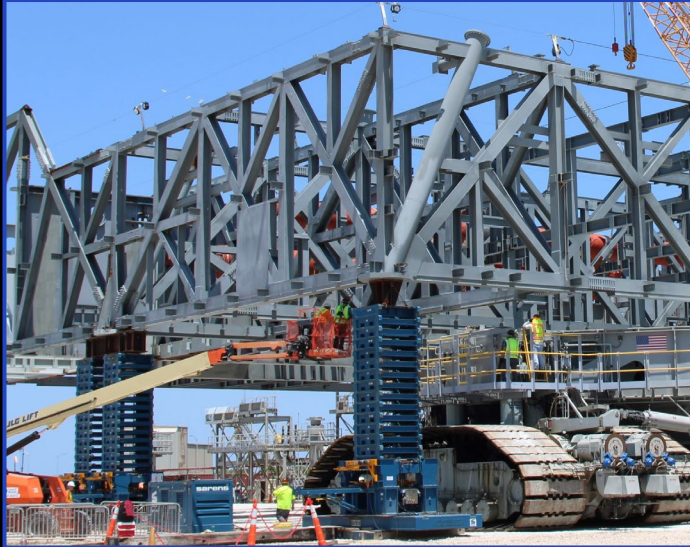
Mobile Launcher 2 'Jack and Set' maneuver
