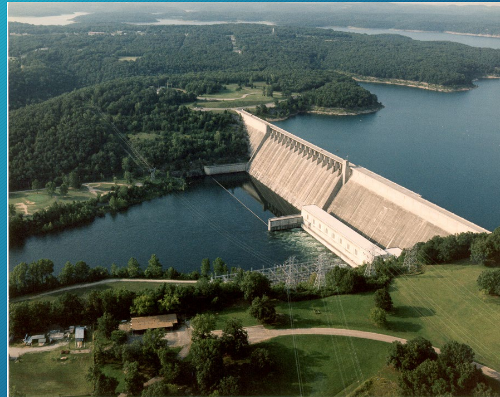
Bull Shoals Dam & Powerhouse, Arkansas (391 MW)
