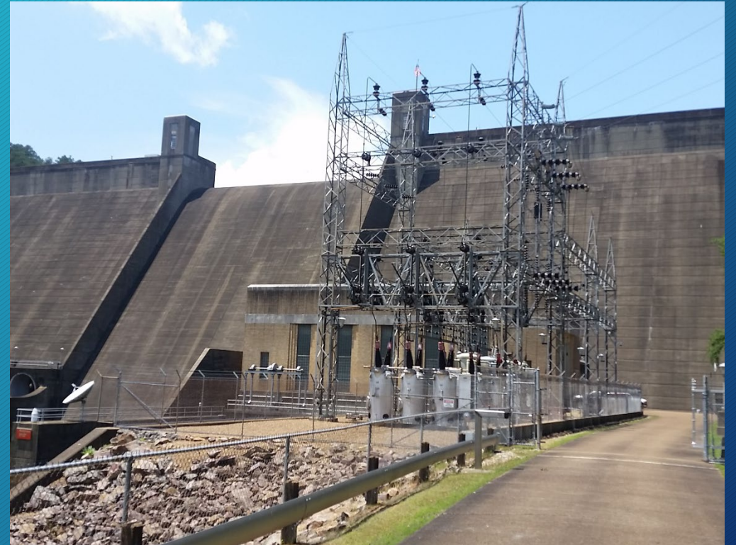
Narrows Dam & Powerhouse, Arkansas (26 MW)
