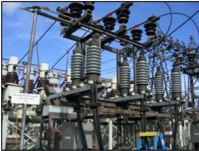
Upgrade 4.8 kV Feeder
