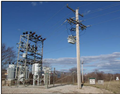
Upgrade 34.5 kV Lines
