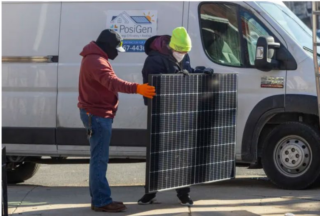
PosiGen employees, Eric Cwiklinski (left) and Tim Miller, prepare to install solar panels on the home of
