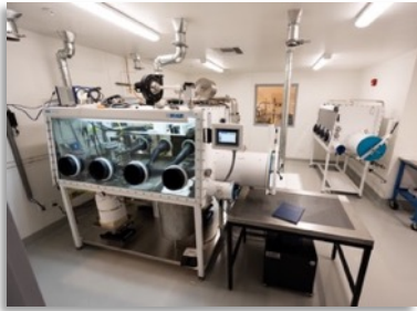
S-Lab Flibe Chemistry and Materials Testing Lab
