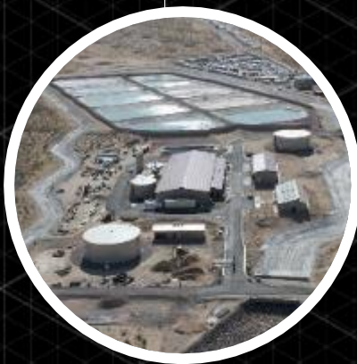
Ft. Irwin, CA Water Treatment Plant
