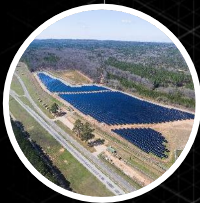
Anniston Army Depot Solar Array
