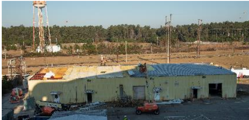
Ongoing Demo 484-4D
