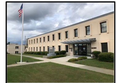
SRNL's Main Building
