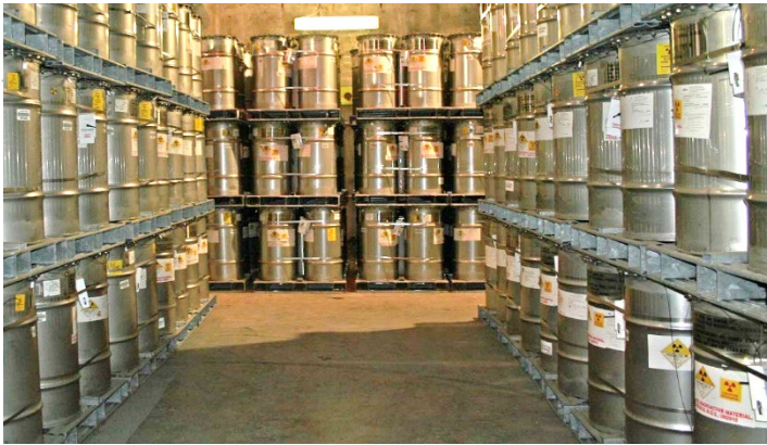
Storage in K-Area
