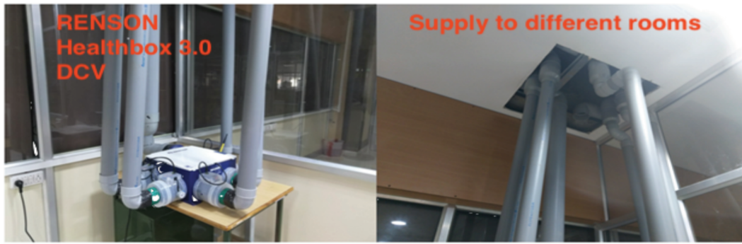
fig. 5.5 Device used for Hybrid Ventilation - Renson Healthbox.
