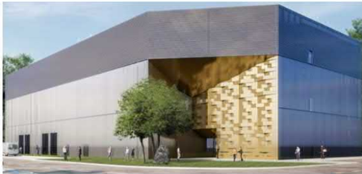
New Preveessin (FR) Computing Center
