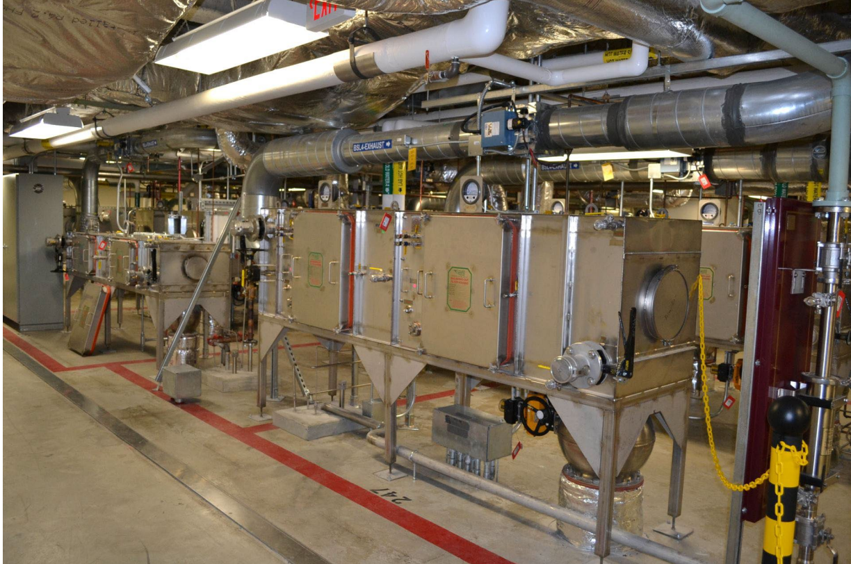
HEPA filtration deck for BSL-4
