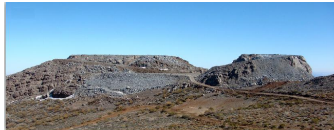
Initial site excavation has created level platforms for the main LSST telescope (L) and calibration telescope (R), while also verifying the required high structural strength of the rock.
