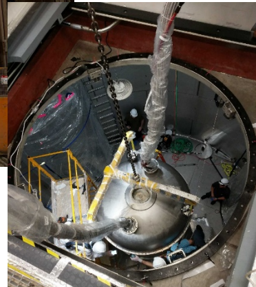
TPC/ICV inside OCV in water tank (Dec. 2019)
