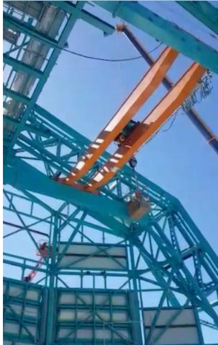
Provisional bridge crane installed and load tested
