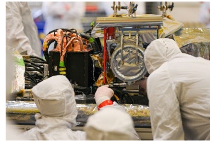
CCOR-1 integration onto GOES-U
