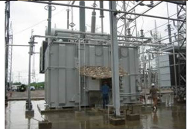
Power Transformer with Installed GIC Monitor and Internal Temperature Sensors
