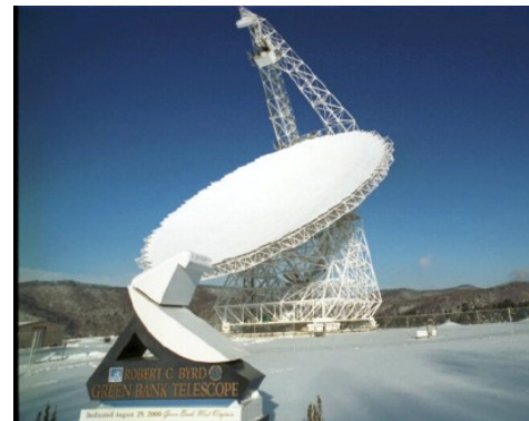
Green Bank Telescope (GBO) 100 m antenna, receive-only
