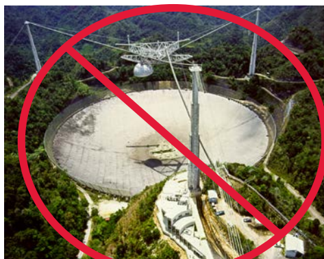
Arecibo (NAIC) 300 m antenna, 1 MW transmitter, 13 cm wavelength (S band)
