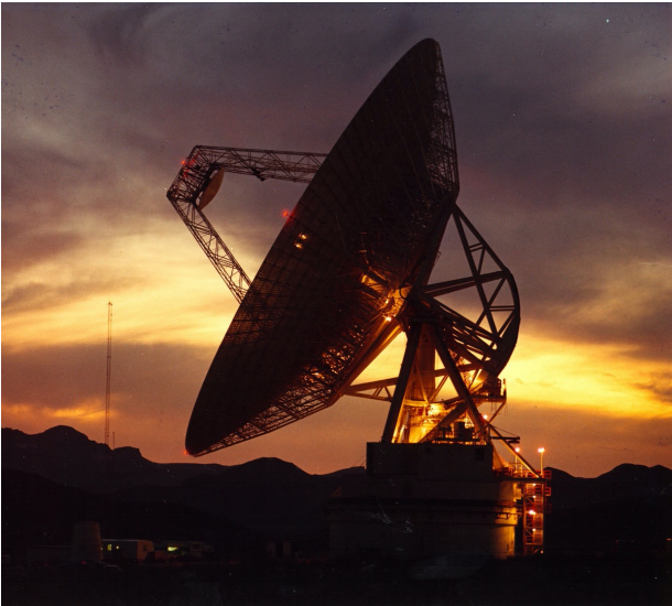
Goldstone Solar System Radar (DSN) 70 m antenna, 450 kW transmitter, 4 cm wavelength (X band)
