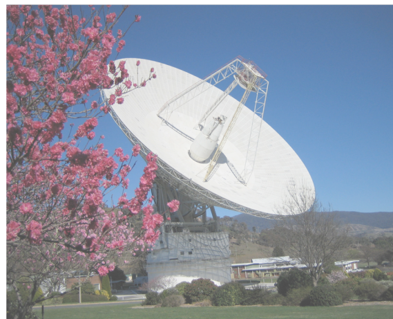
Canberra DSS-43 (DSN) 70 m antenna, 80 kW transmitter, 4 cm wavelength (C band) + Australia Telescope Compact Array
