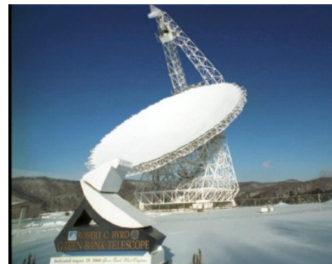
Green Bank Telescope (GBT) 100 m antenna, receive-only
