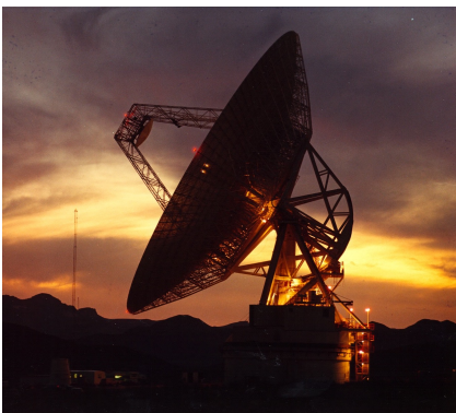
Goldstone DSS-14 (DSN) 70 m antenna, 500 kW transmitter, 4 cm wavelength (X band)
