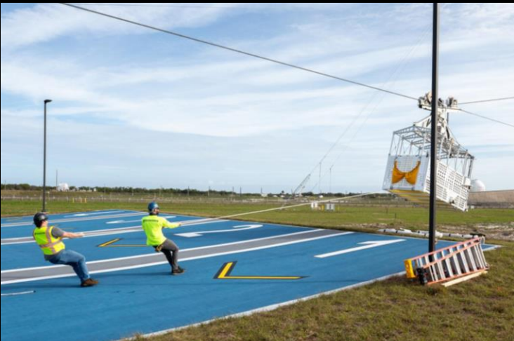
In preparation for the Artemis II crewed mission, EGS teams begin installation of four emergency egress baskets at Launch Complex 39B
