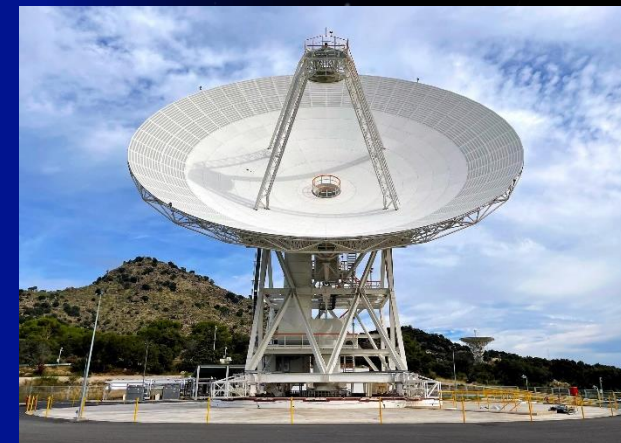
Deep Space Station 53 is a new waveguide antenna that went online in February 2022 at NASA's Deep Space Network's ground station in Madrid.
