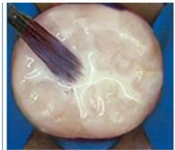
Painting Sealant into Grooves
