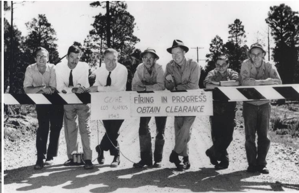
One of multiple explosives firing sites, 1945
