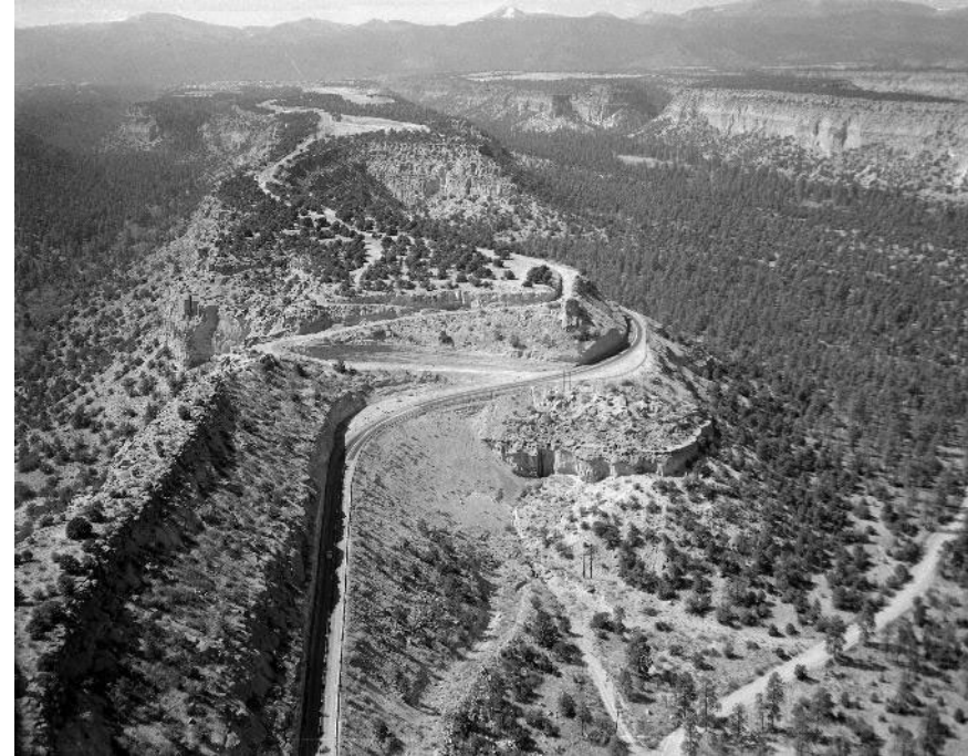
Main Hill Road with original switchbacks (middle) and wartime bypass (right).
