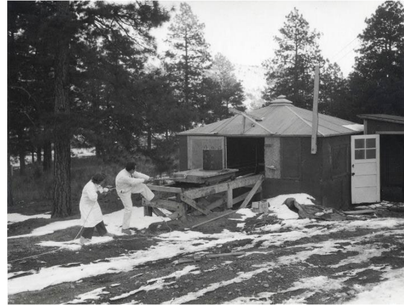
Wartime "remote handling" of a kilocurie source of radiolanthanum for RaLa testing, Bayo Canyon (TA-10)
