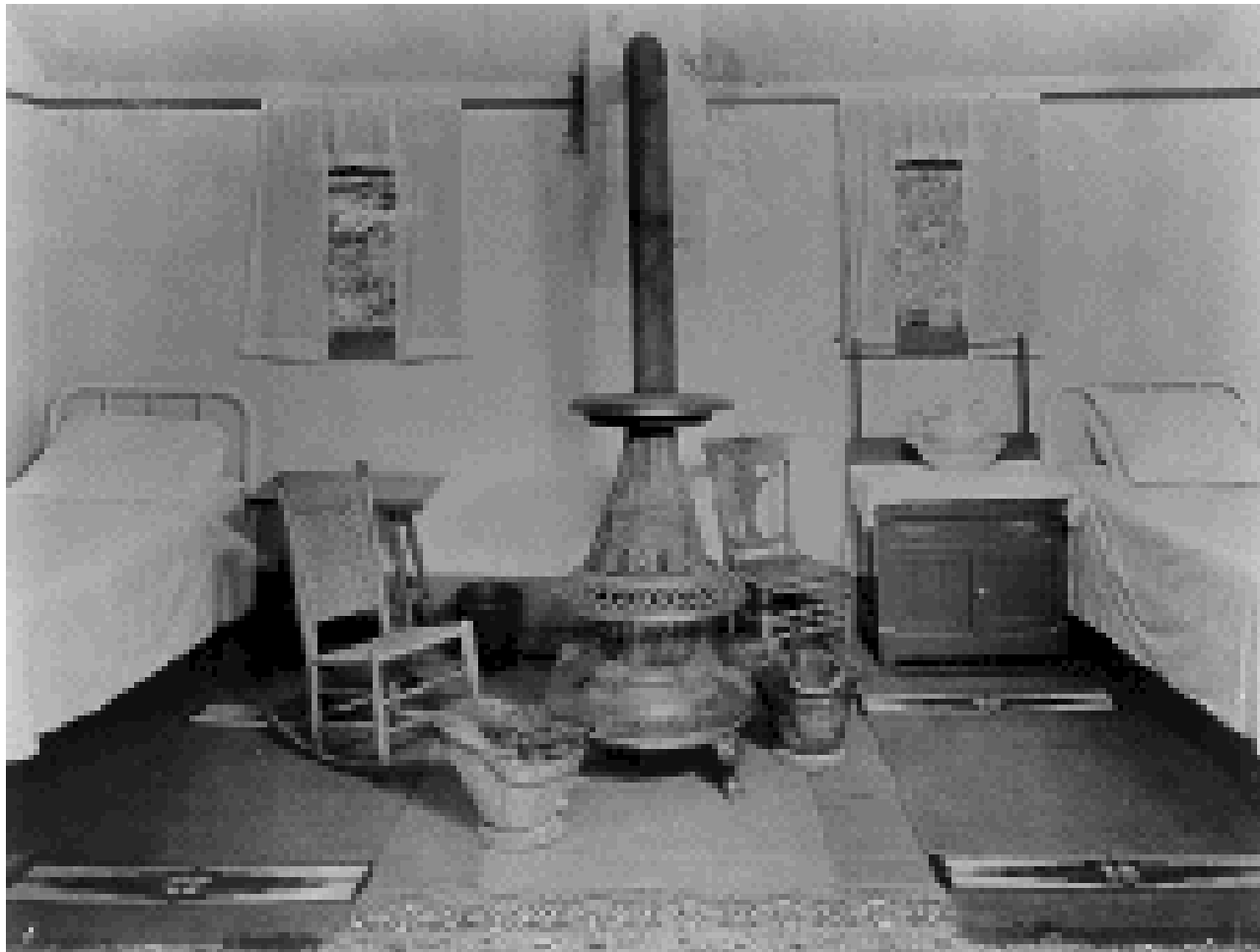
Interior view of “Little Red” New York 1884
